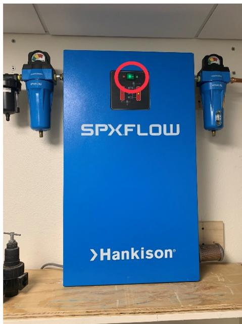
3. Slowly turn on the main air. The action should take about 10-20 seconds. Confirm at the pressure gage near the instrument that air flow is 60-80 psi.
