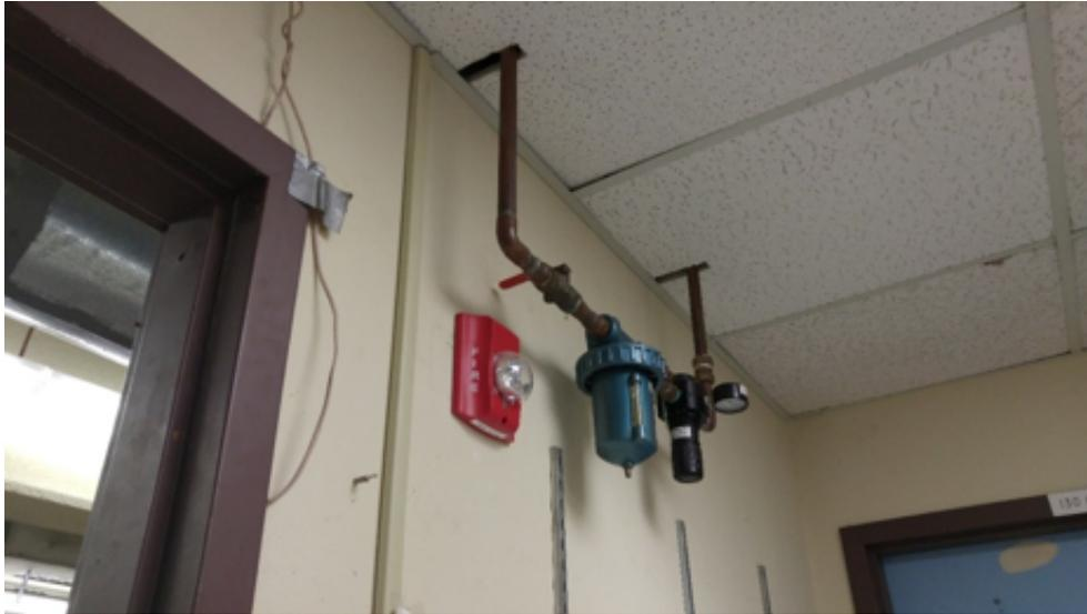
*Off: the red handle is perpendicular to the pipes*
